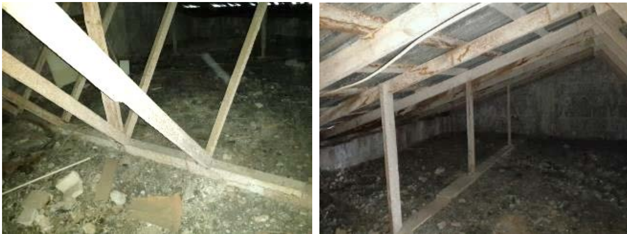
Figure 7: Wooden timber-frame of the roof and asbestos and/or metal sheeting
