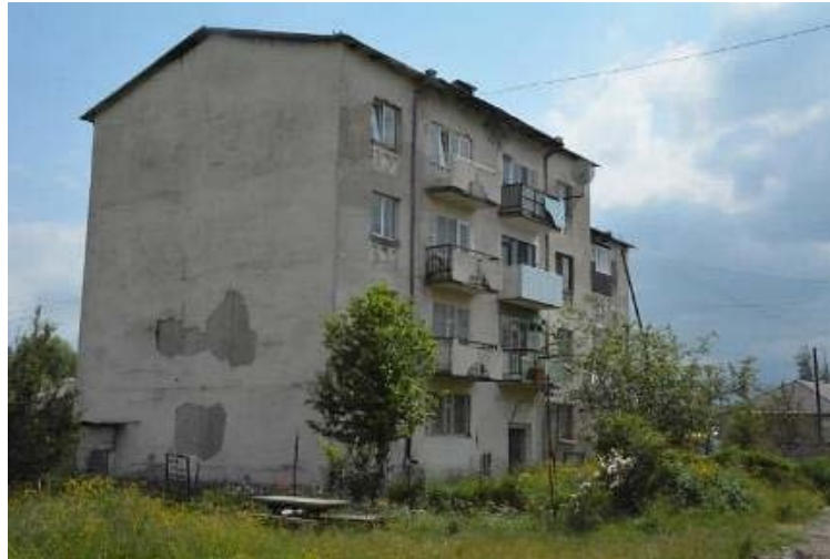
Figure 6: External walls of the residential buildings made with reinforced concrete
