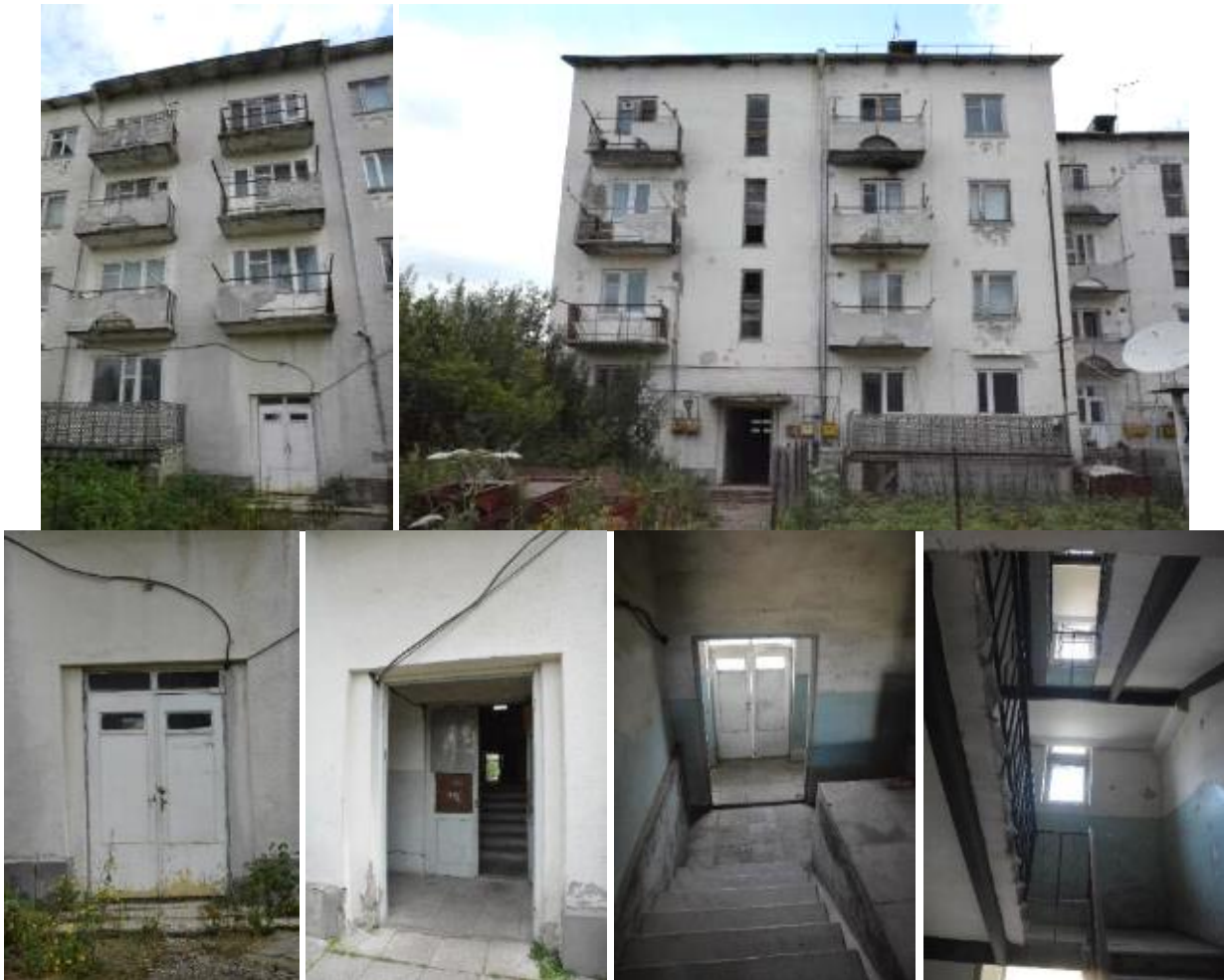
Figure 8: The entrance doors and windows of the buildings
